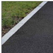
Tarmac path with pin kerb edge
