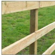
Post and rail fencing
