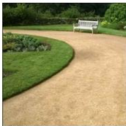
Self binding gravel with timber edging
